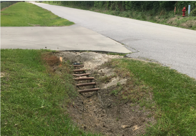
Repair storm drainage infrastructure near park roads.
