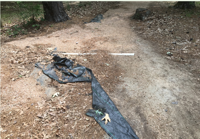
Maintain path surface to provide an adequate walking or riding surface free from obstacles and hazards.
